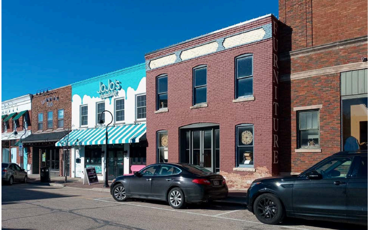
Beidelman "Workshop" in context with neighboring buildings 2024—Naperville Preservation, Inc.
