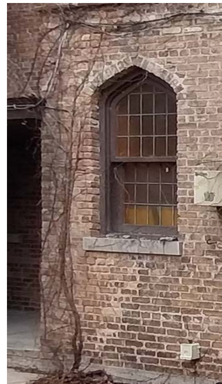
Mortuary window, 2024 —Naperville Preservation, Inc.
