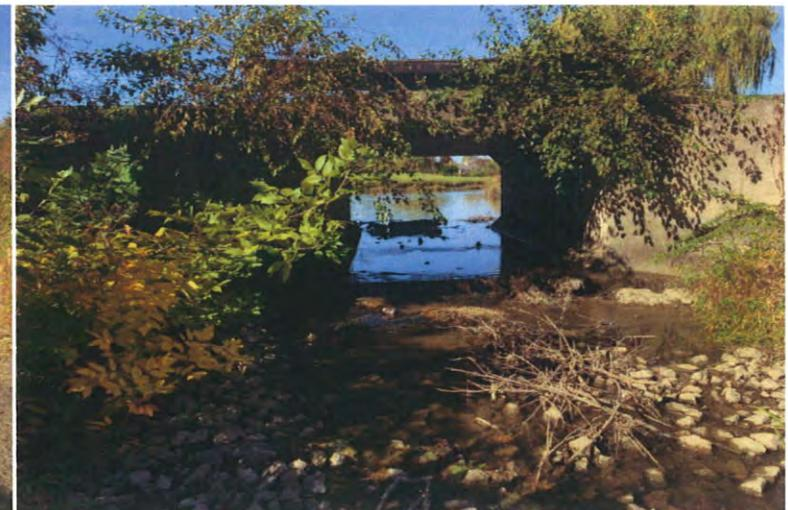
A concrete weir and box culvert was observed within Clow Creek on the West property line.
