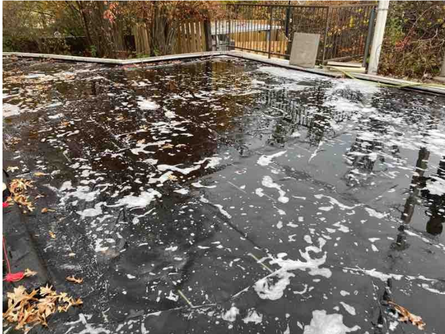
West Overview of Area 1.0 - Section 1
