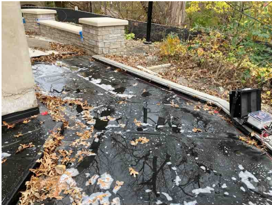
West Overview of Area 1.0 - Section 1
