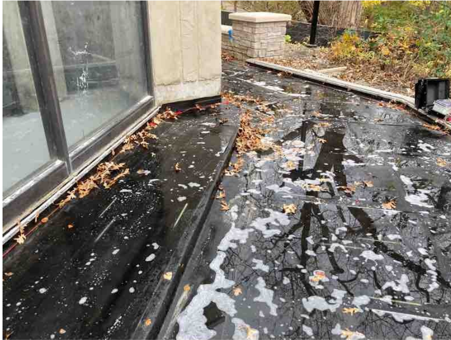
West Overview of Area 1.0 - Section 1
