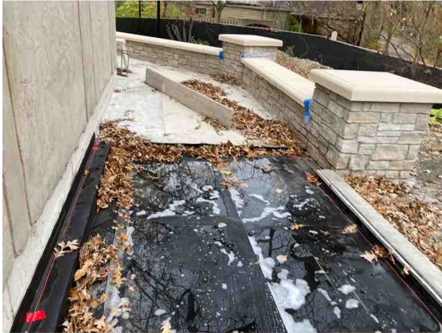
West Overview of Area 1.0 - Section 1
