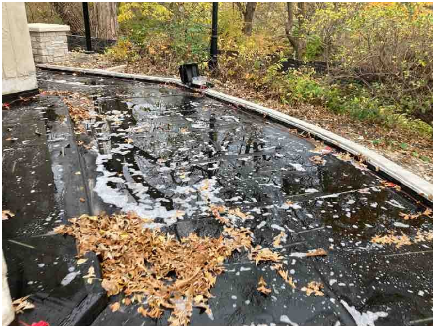
West Overview of Area 1.0 - Section 1
