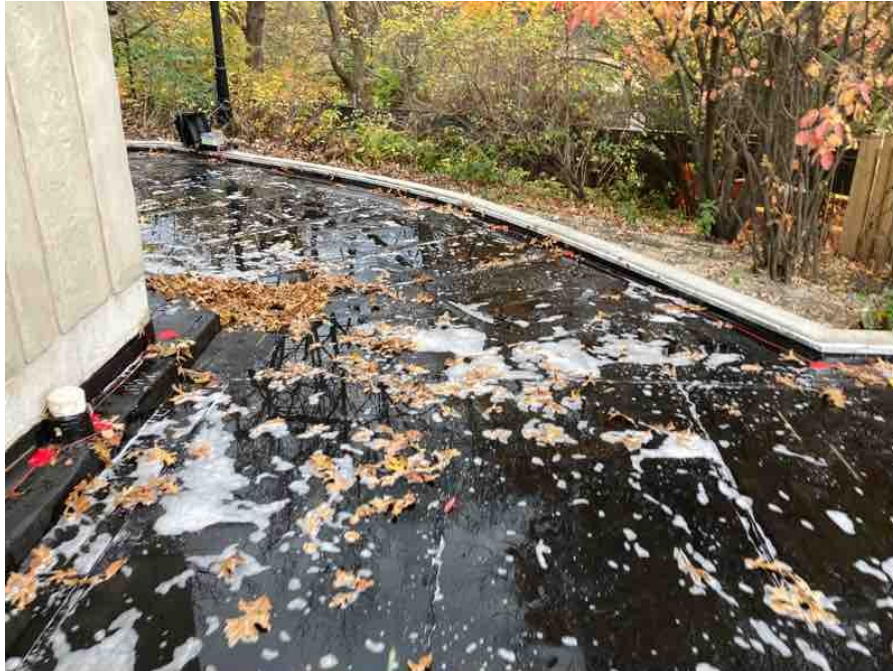
West Overview of Area 1.0 - Section 1
