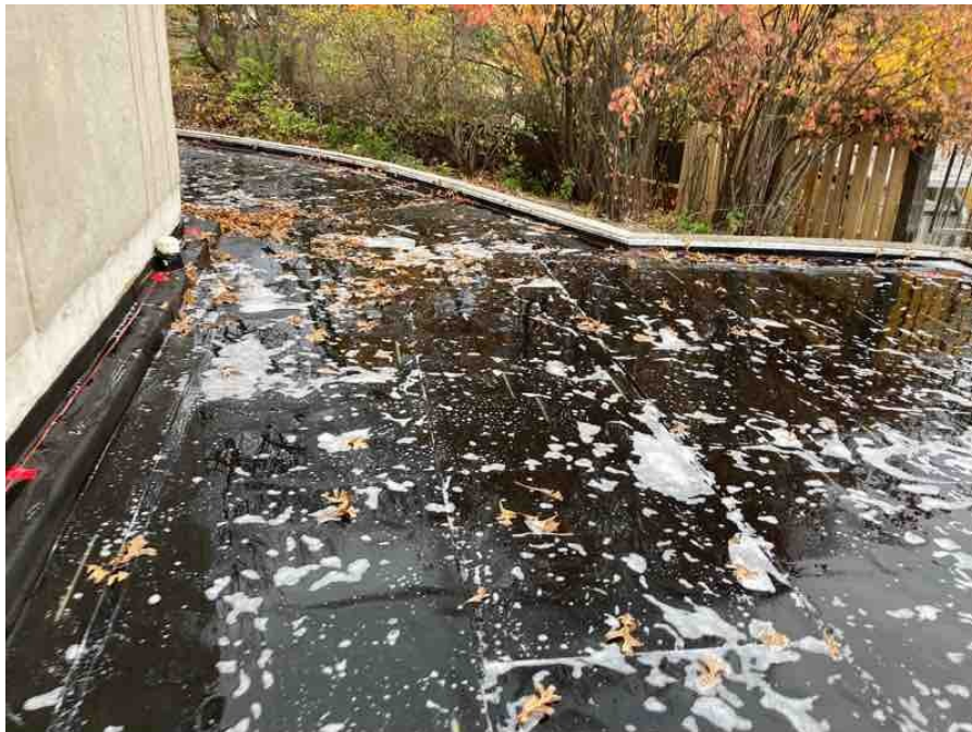
West Overview of Area 1.0 - Section 1
