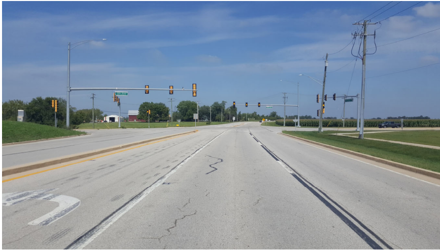
Northbound Plainfield-Naperville Rd (119 th St intersection)
