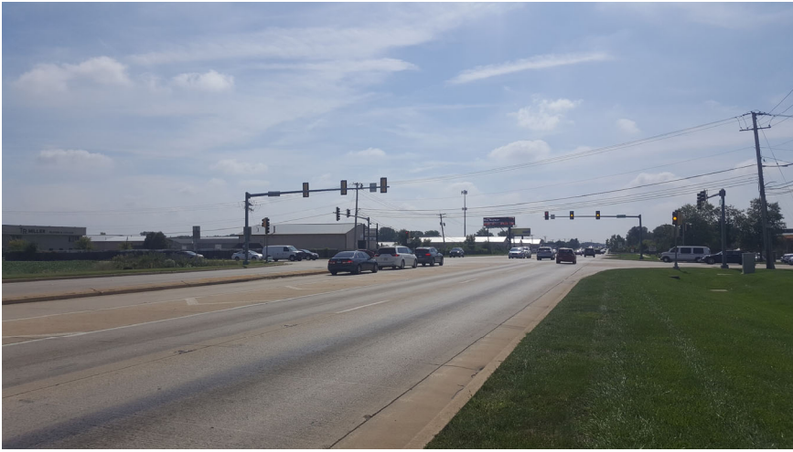
Southbound IL 59 (119 th St intersection)
