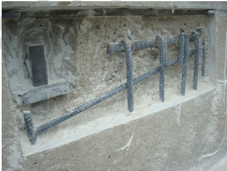
Photograph #3: Exposed end of PT rod and reinforcement bars at right opening
