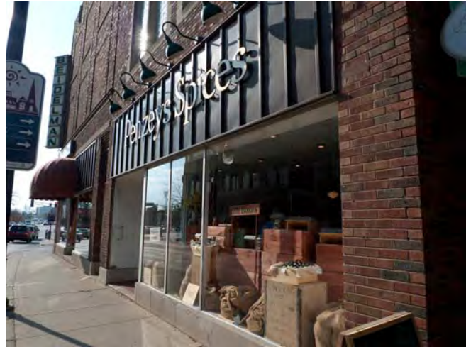
Storefront level at east elevation
