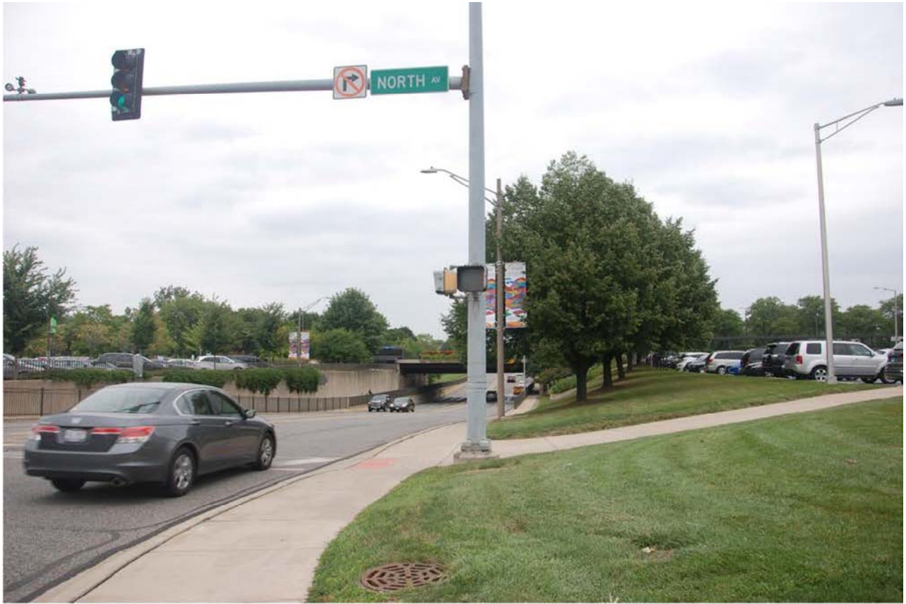
Figure 8: Washington at North looking north toward the underpass – Current
