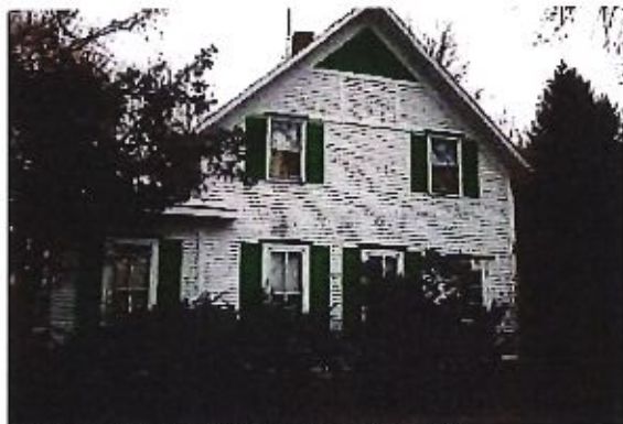
Existing Farm-Style Home proposed to be demolished
