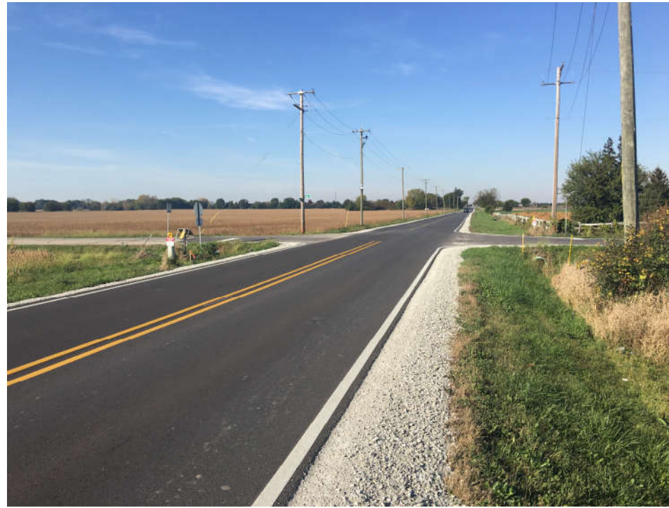
Looking west along 119 th St at Book Rd
