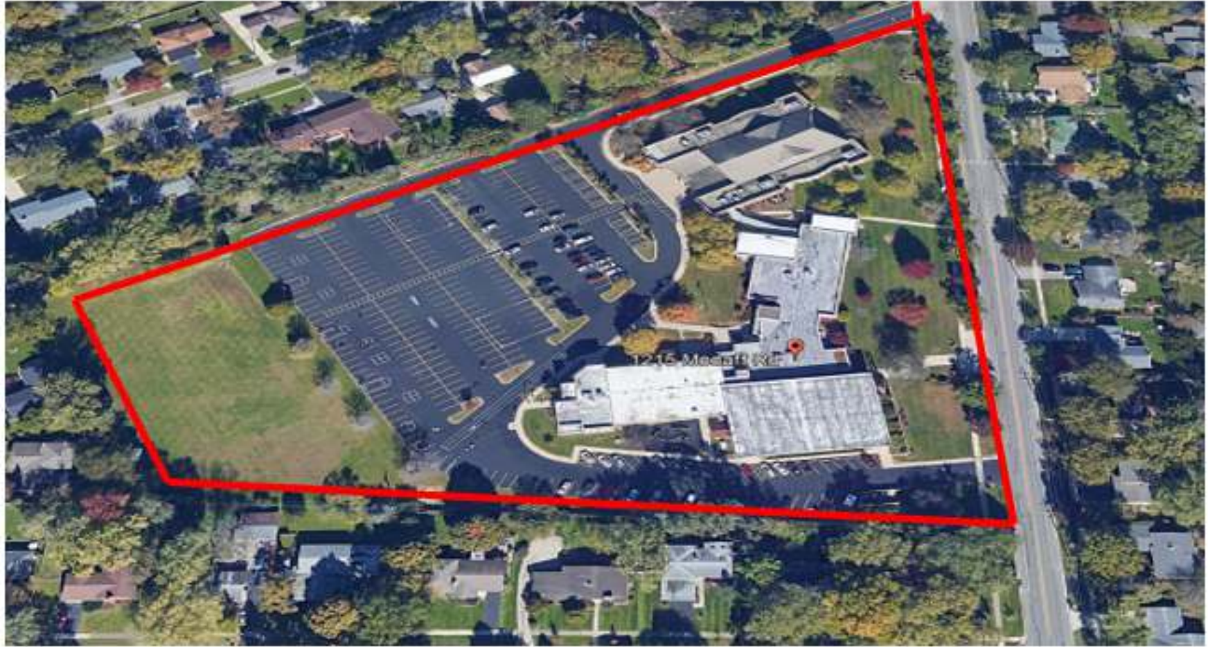
St. Raphael Church and School (Grades K-8) 1215 Modaff Road, Naperville
