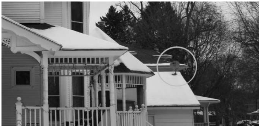
Photo D.29 - Encouraged satellite dish placement
