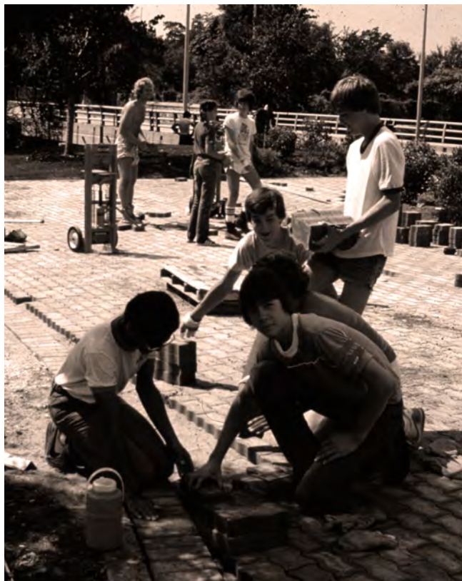
Volunteers Lay Bricks - 1981
