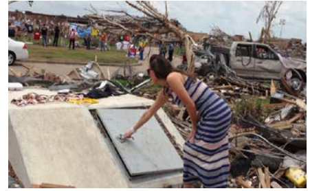
Exhibit 5-5 Tornado Safe Room
