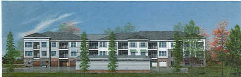
3. SOUTH ELEVATION - SHOWING DETACHED GARAGES
