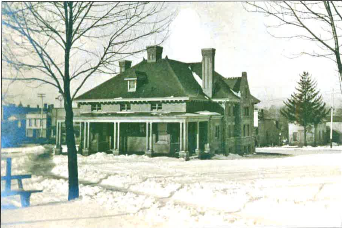
East and North Facades Looking Southwest (n.d.)
