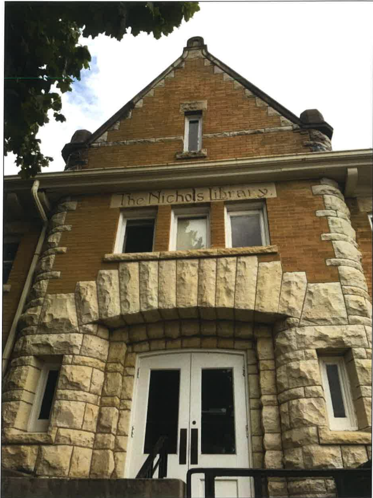
Main Entrance (May 2017)
