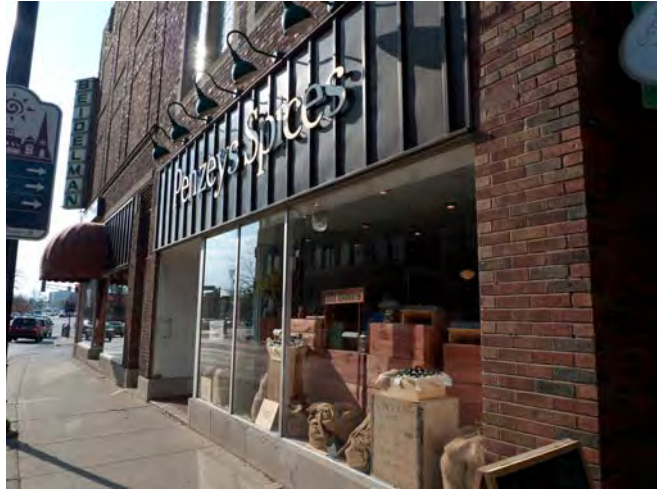
Storefront level at east elevation
