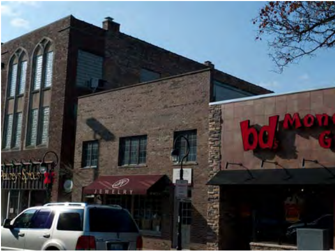
Partial north elevation
