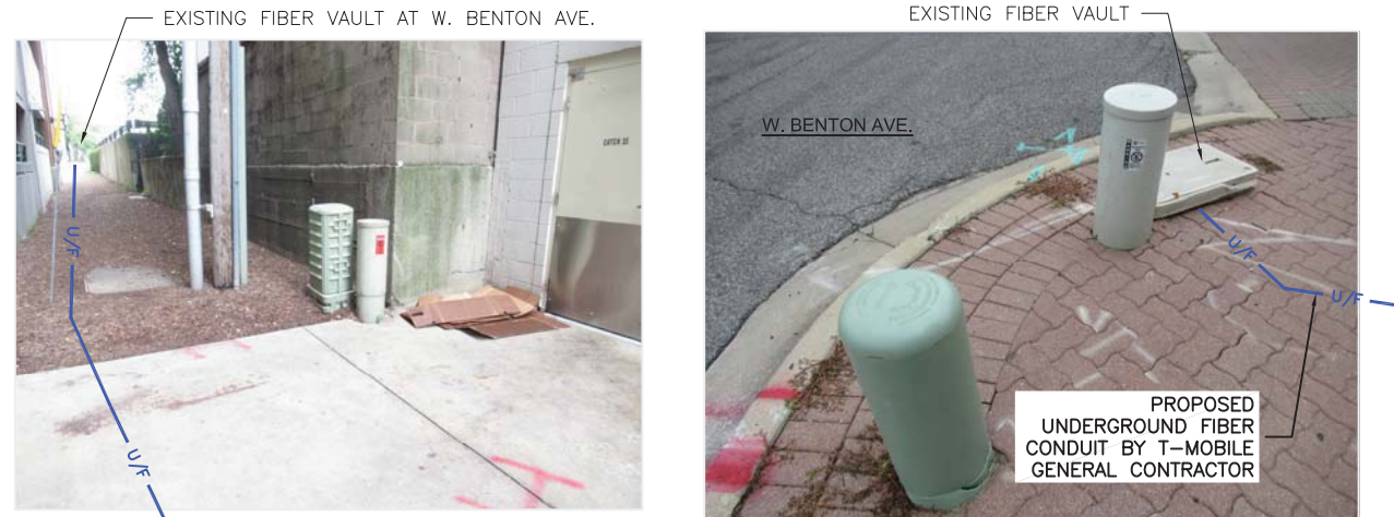
PROPOSED ROUTE OF UNDERGROUND FIBER CONDUIT ALONG RIGHT-OF-WAY.
