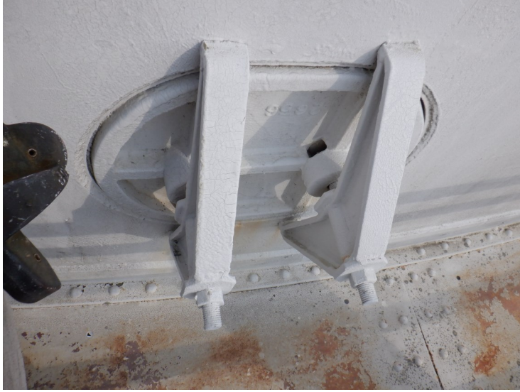
34) The sidewall manway is in good condition.
