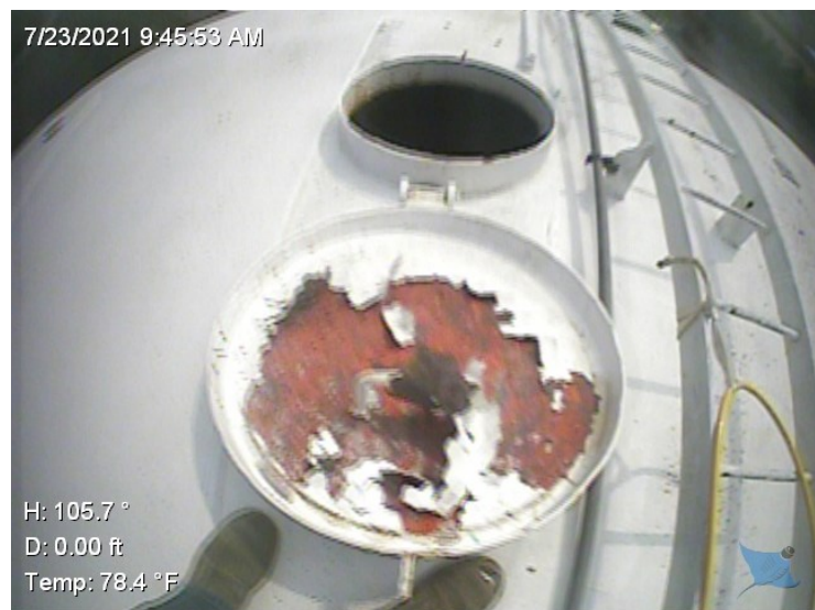
50) The wet interior roof hatch is in good condition. There are spot coating failures on the cover.
