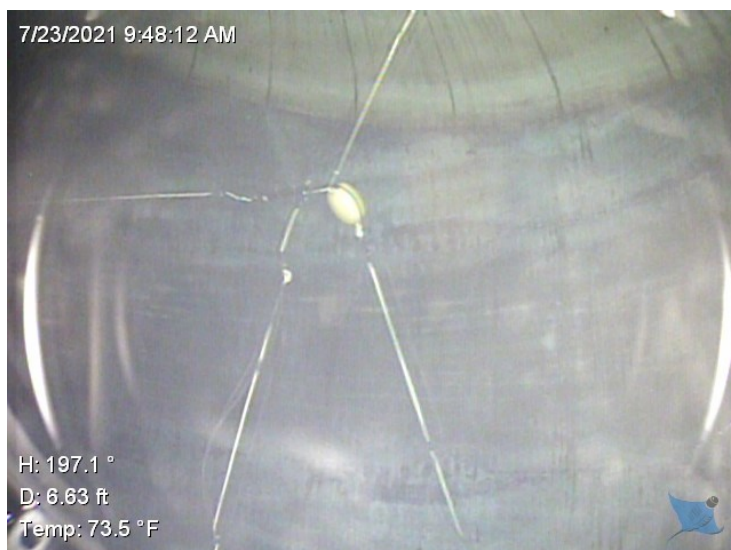
60) The floating ring cathodic protection system appears to be in good condition.
