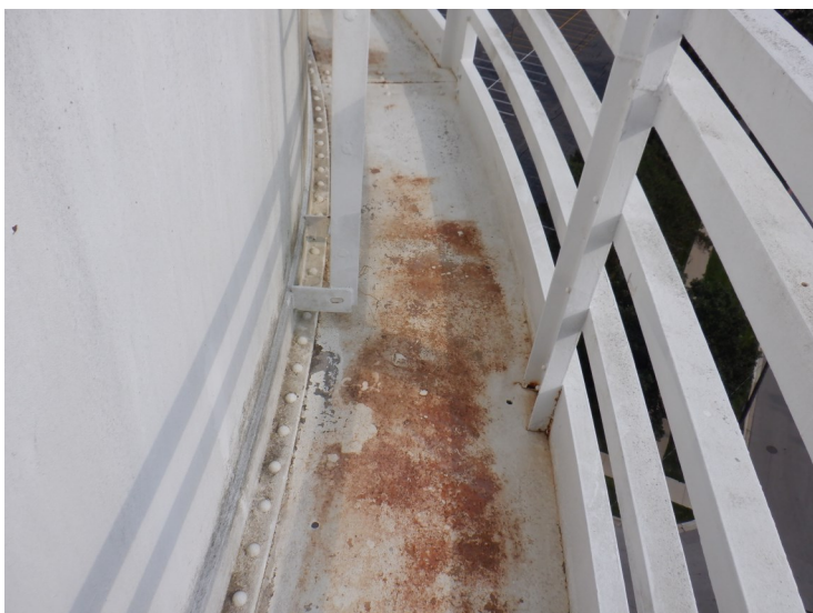
30) The balcony is in good condition. The coating is in poor condition.
