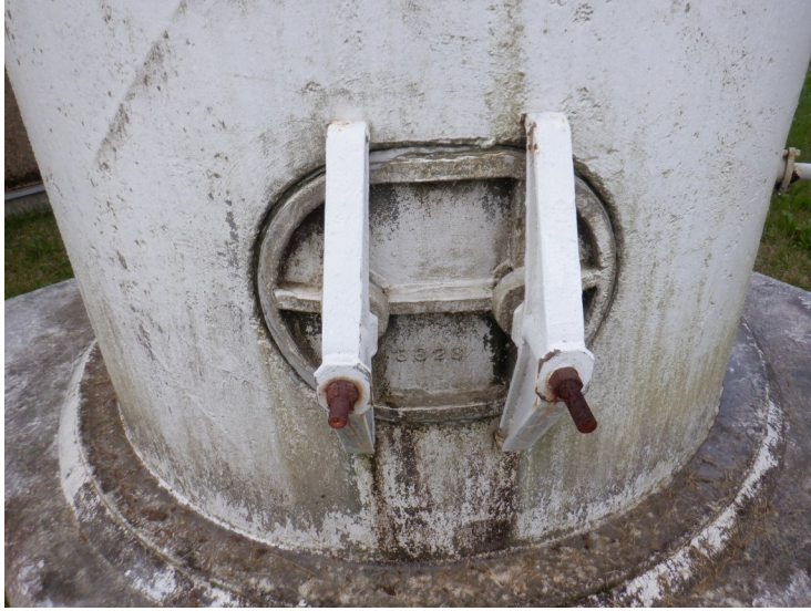
4) The elliptical riser manway is in good condition.
