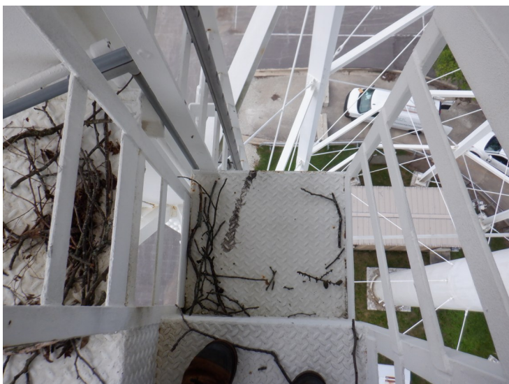
24) The step-off platform under the bowl is in good condition. There are remains of a hawk nest on the platform.
