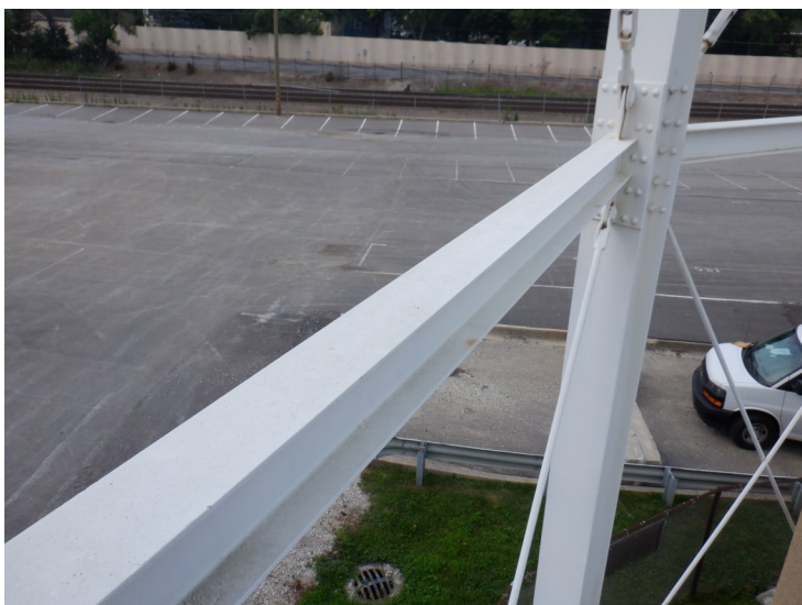
21) Typical strut section that is in good condition. The coating is in fair condition overall.
