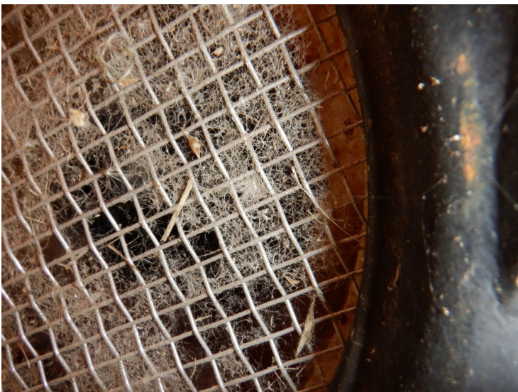
15) The overflow pipe screen is in good condition.
