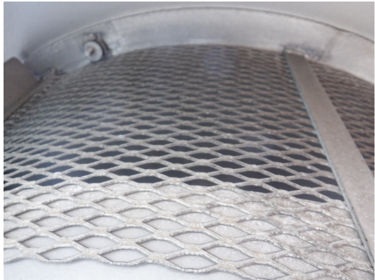
41) The outer vent screen is in good condition.
