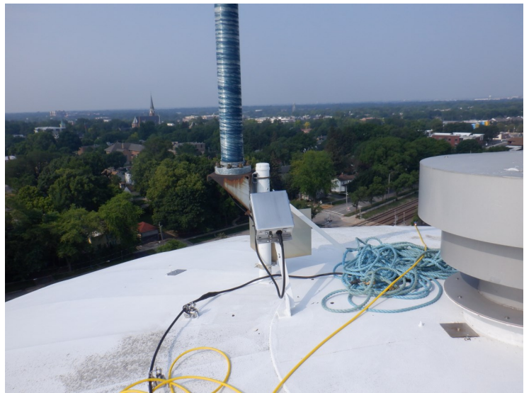
44) There are antennas on the roof.
