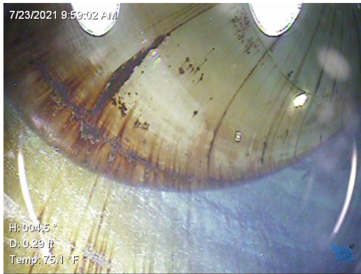
55) Spot coating failures on the wet interior sidewall.
