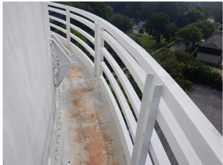
32) The balcony handrail is in good condition.
