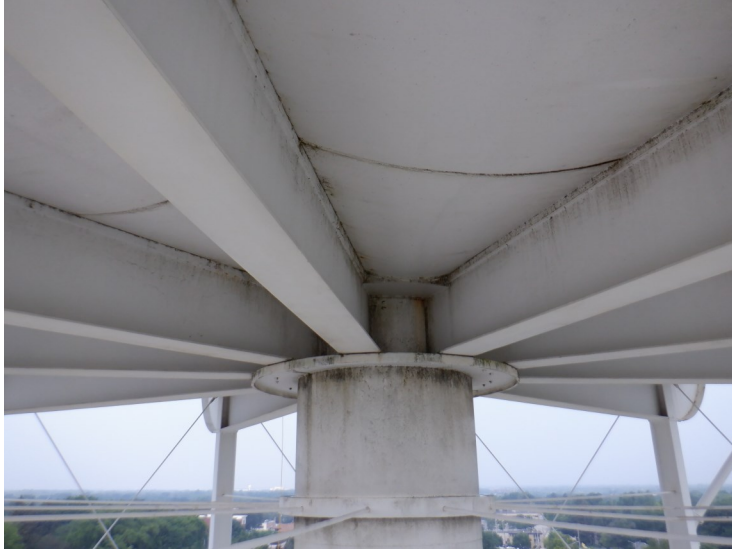
25) The bowl coating is in fair condition overall. There is mildew growth on the bowl.
