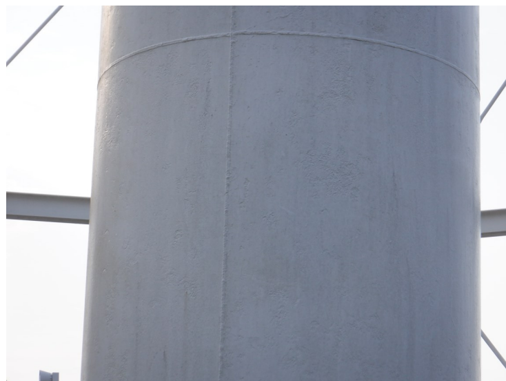
6) The riser coating is in fair condition overall.
