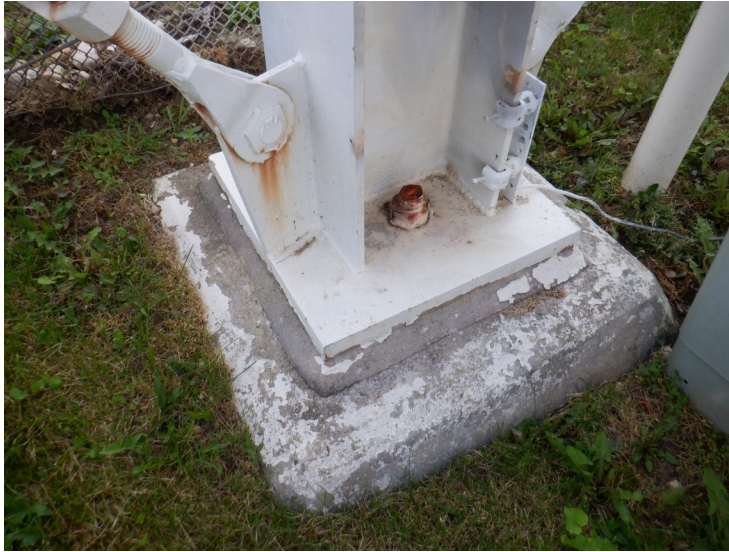
10) Typical leg foundation that is in good condition. The coating is in poor condition overall.
