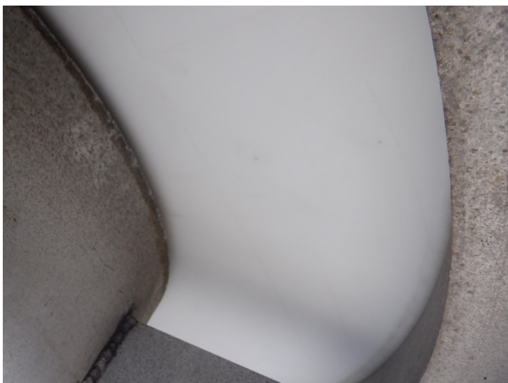
42) The vent pressure plate is in good condition and was found to be properly aligned during the inspection.
