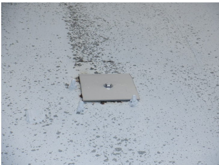
39) Bolted cathodic cover on the roof that is in good condition.
