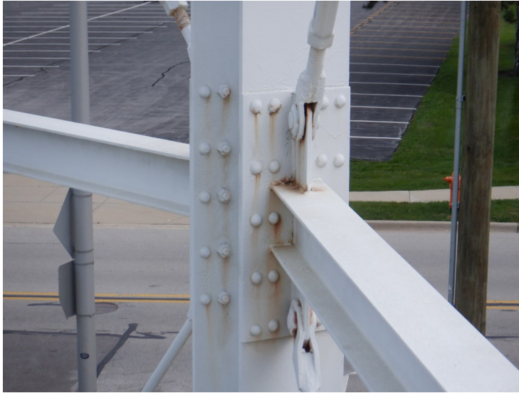
22) Spot coating failures and rust bleedthrough at a strut and leg connection.
