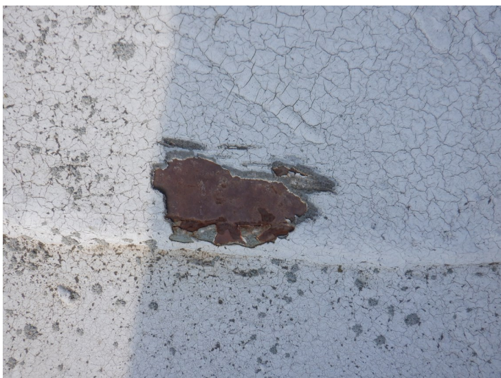
48) Spot coating failure on the roof.
