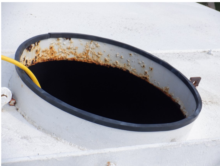
51) A gasket was installed on the wet interior hatch by Dixon during the inspection.
