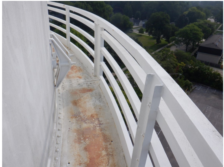
32) The balcony handrail is in good condition.
