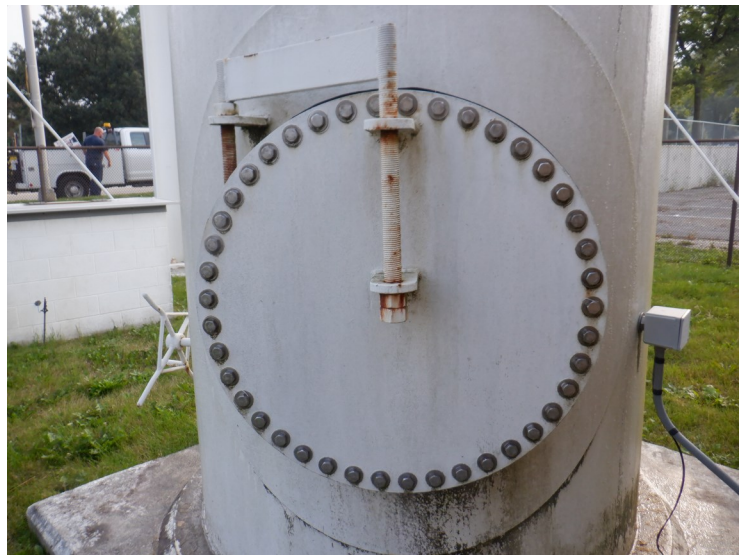
5) The bolted riser manway is in good condition.
