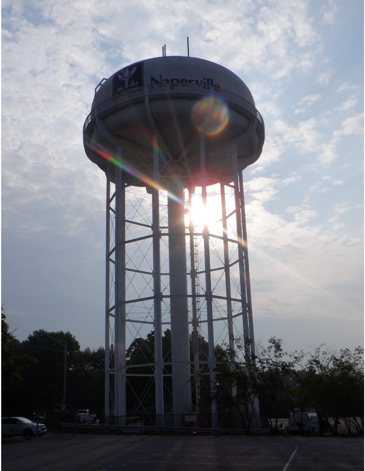
500,000 gallon radial arm (Central Tank) located in Naperville, Illinois.
