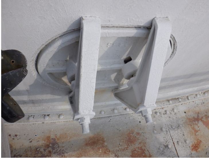
34) The sidewall manway is in good condition.
