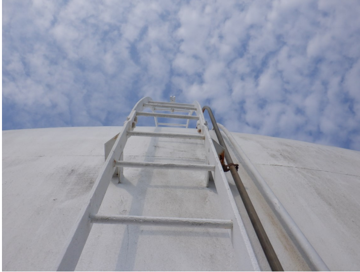
37) The sidewall ladder is in good condition. The ladder is not equipped with a fall prevention device.
