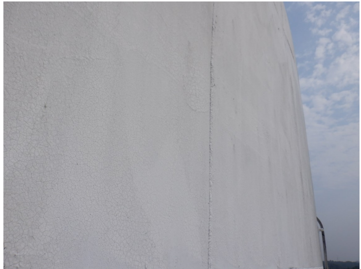
35) The sidewall coating is in fair condition overall.
