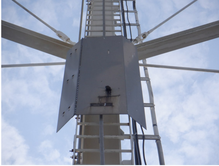
19) The leg ladder is equipped with a vandal guard that is in good condition.
