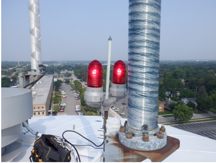
40) The double red aviation light is in good condition.
