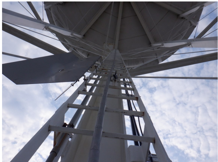
20) The ladder is in good condition. The ladder is equipped with a fall prevention device.
