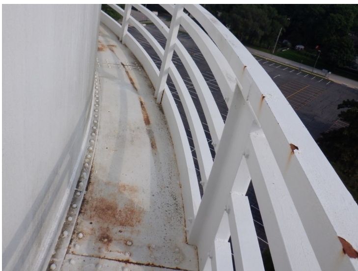
33) Spot coating failures on the handrail.
