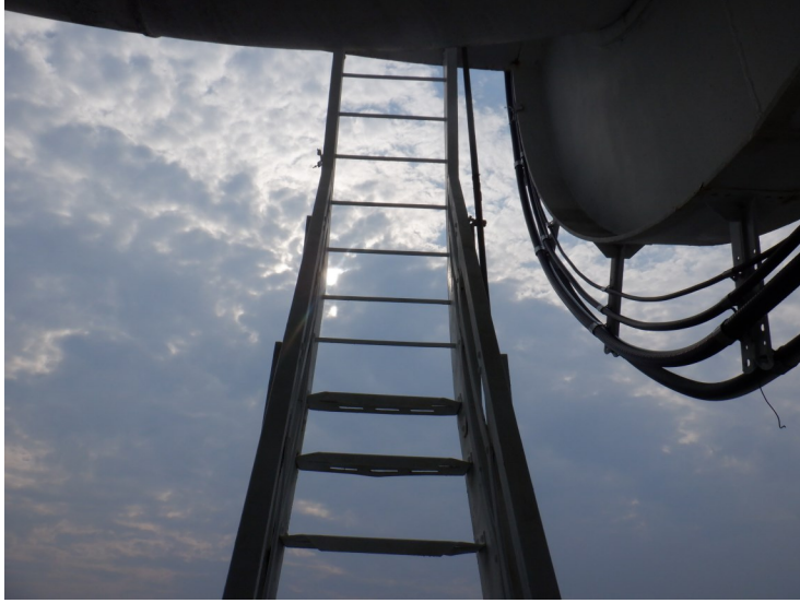
28) The stairs and ladder to the balcony are in good condition.
