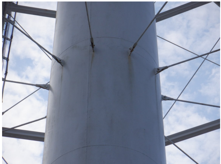
8) The riser tie rods are attached to welded lugs that are in good condition.
