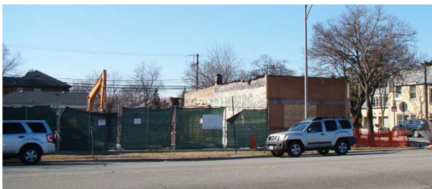
New residential construction is underway at the east corner of North and East Avenues.
