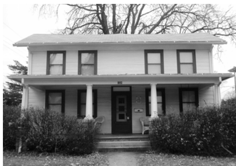
Photo C.15 - I-Form vernacular style residence - 154 Center Street
