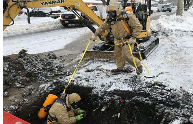
Repairing damage caused by water main break
