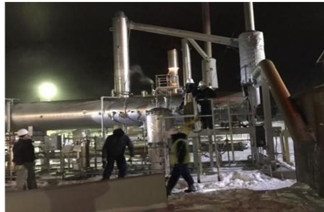
Storage reboilers are critical in maintaining gas quality during withdrawals
