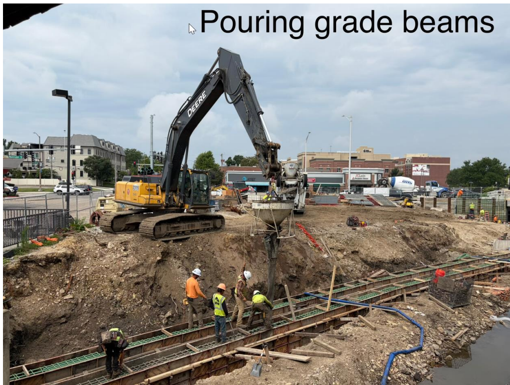
Pouring the concrete grade beams for the low flow walk at the southeast corner of the site
