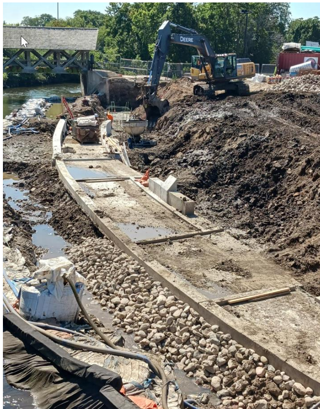
Low flow concrete slab at the northwest corner of the site
