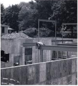
PRE-EMPTION HOUSE CONSTRUCTION
