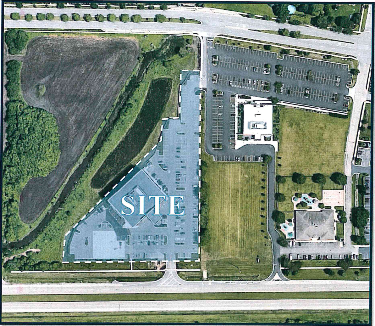
Aerial View of Site
