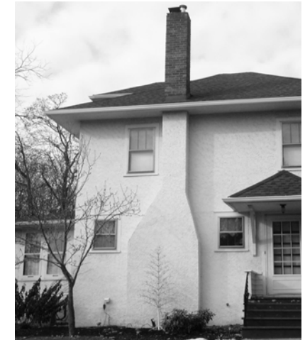
Photo D.7 - Stucco house with brick chimney - 125 S. Columbia Street
