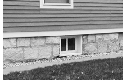
Photo D.4 - Limestone foundation wall
