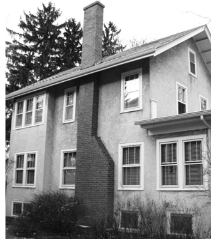
Photo D.6 - Stucco house with brick chimney - 141 N. Brainard Street
